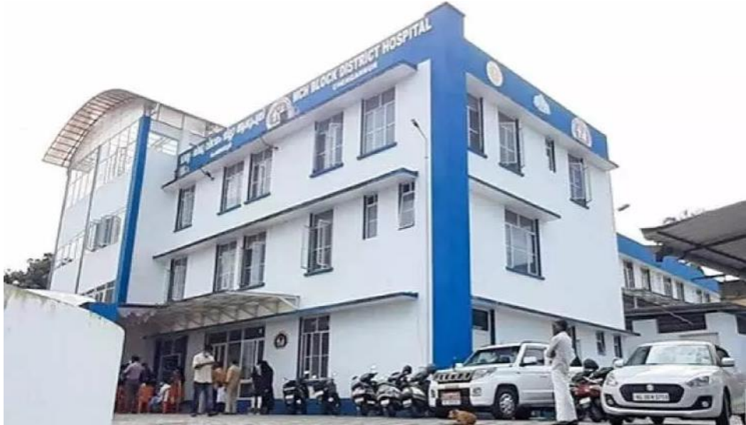
Figure1.5. District Hospital Chengannur
